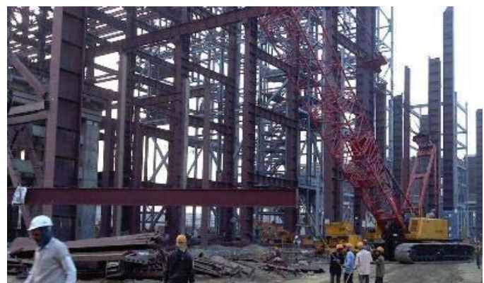
SOME IMAGES OF STEELSTRUCTURES
