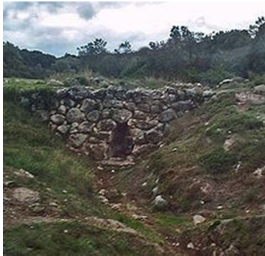
Fig 1: The Arkadiko Bridge in Greece (13th century BC), one of the oldest arch bridges in existence
