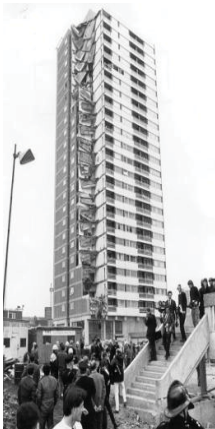
Fig.1. Ronan point after collapse.
