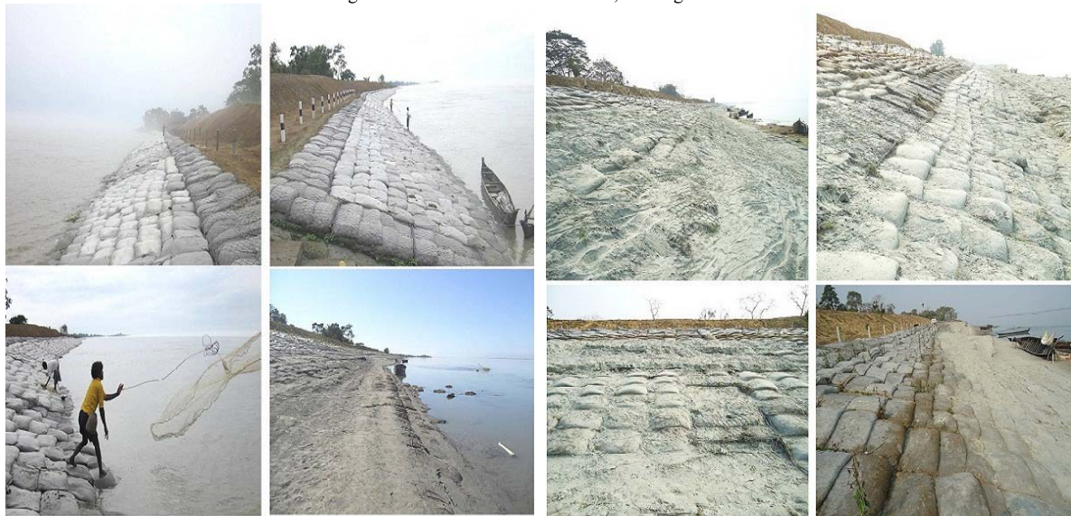
Figure 6. Bank condition during flood
