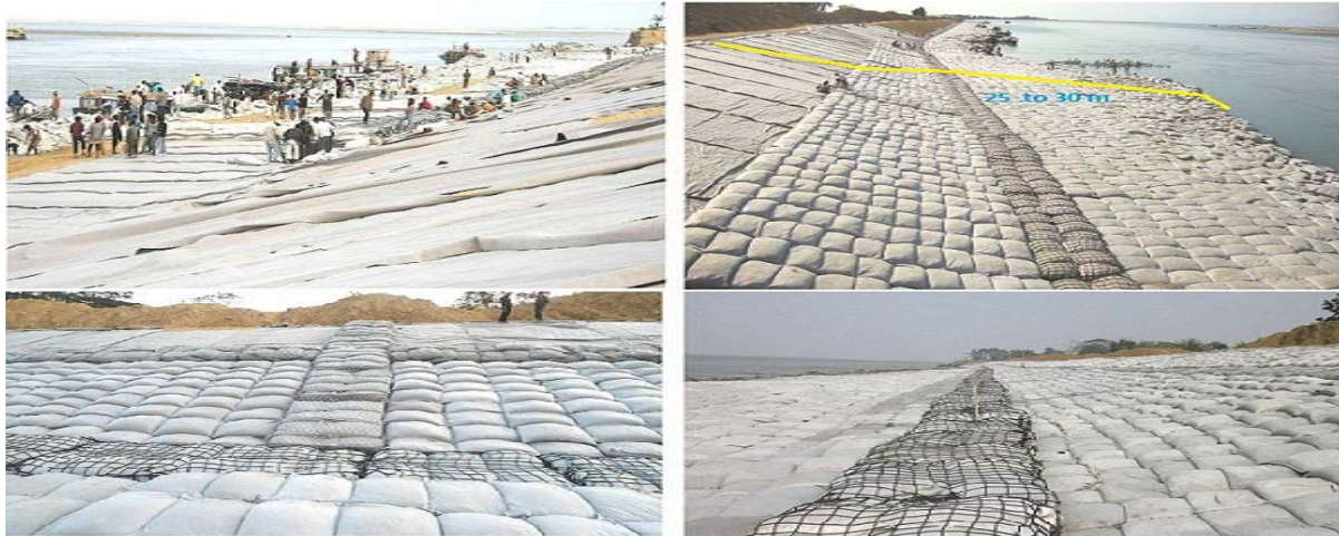
Figure 5. Placement of filter media, Geobags & PP Gabions
