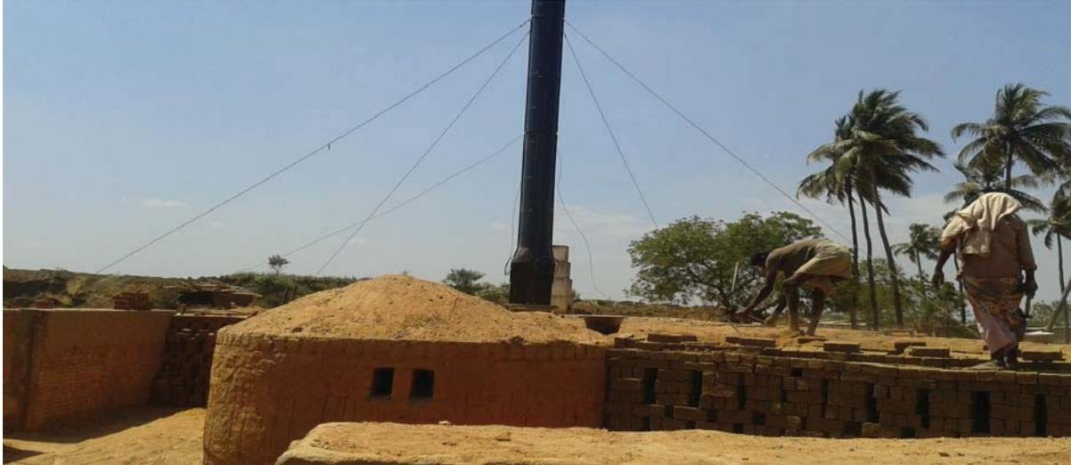
Fig7: Firing of bricks in the clamp
