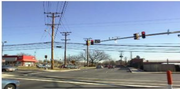
Figure 6. Diagonal Mast-Arm Installation
