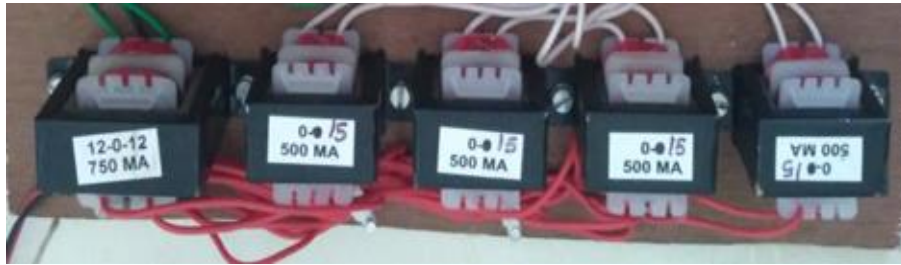
Picture1: There are 5 Transformer one is for microcontroller and remaining 4 is for TLP250
