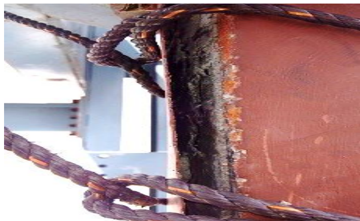
Fig 11. Local failure of column 1 without connectors
