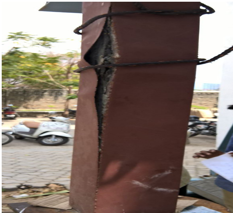
Fig 13. Local failure of column 2 with connectors
