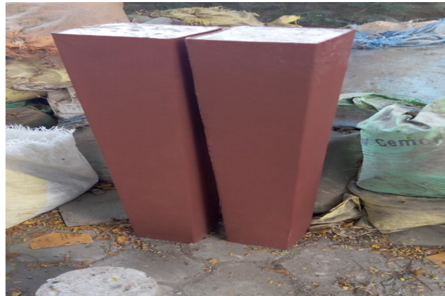
Fig 6: Columns painted with red oxide
