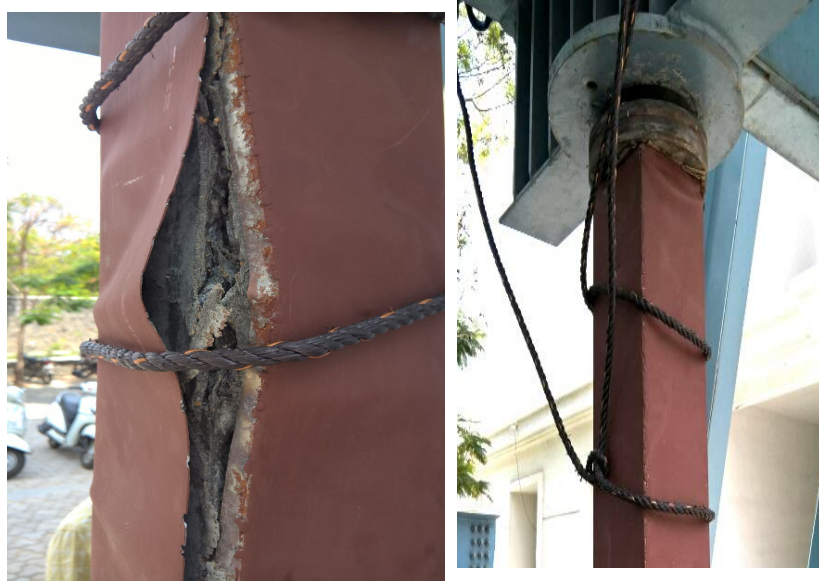
Fig 14. Local failure of column 2 with connectors
