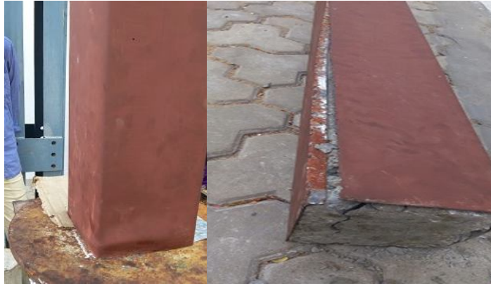
Fig 12: Local failure of column 1 without connectors
