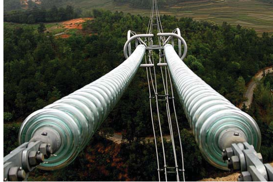
FIG.2: Glass Insulator String For High Voltage Overhead Transmission Line
