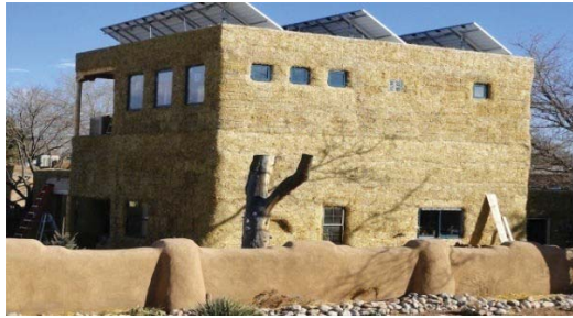
Fig. 1: Load Bearing Straw-bale Walls
