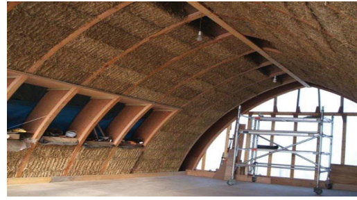
Fig. 2: Non Load Bearing Straw-bale Walls
