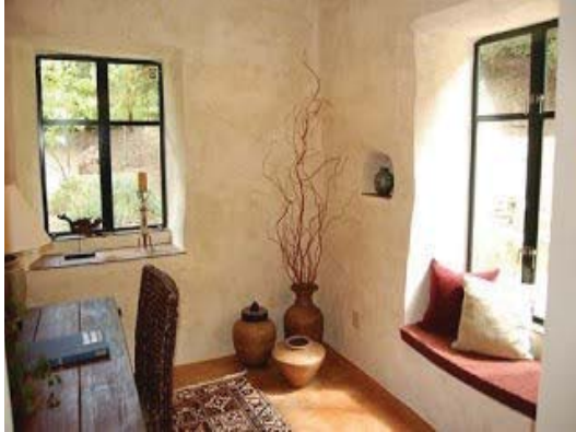
Fig. 4: Sand Base Plaster
