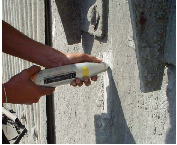
Rebound Hammer Test
