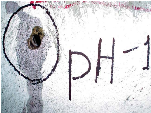
Carbonation of Concrete
