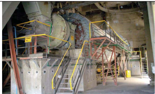
Foundation Tail End
