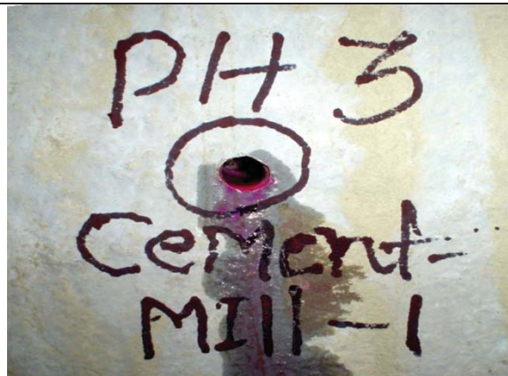
Carbonation of Concrete
