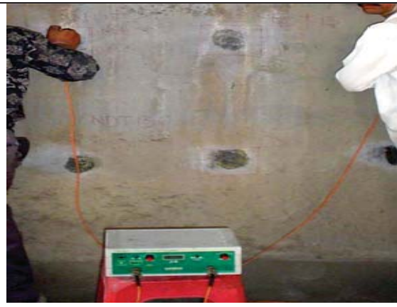
N.D.T. of structure
