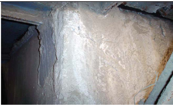
Damaged Tail End
