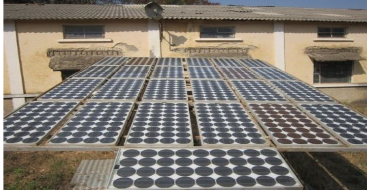
Fig.1 Photovoltaic system at Ujjain Engineering College, Ujjain (M.P.)-India.
