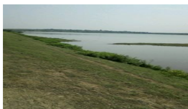
Figure no. 03 Photo of Narawala Reservoir
