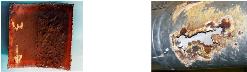
Fig. 1: Typical Corrosion in Pipe
