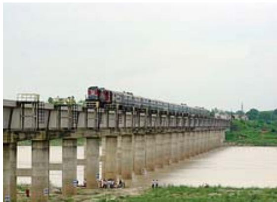
Fig. 7 Train is on River Bridge
